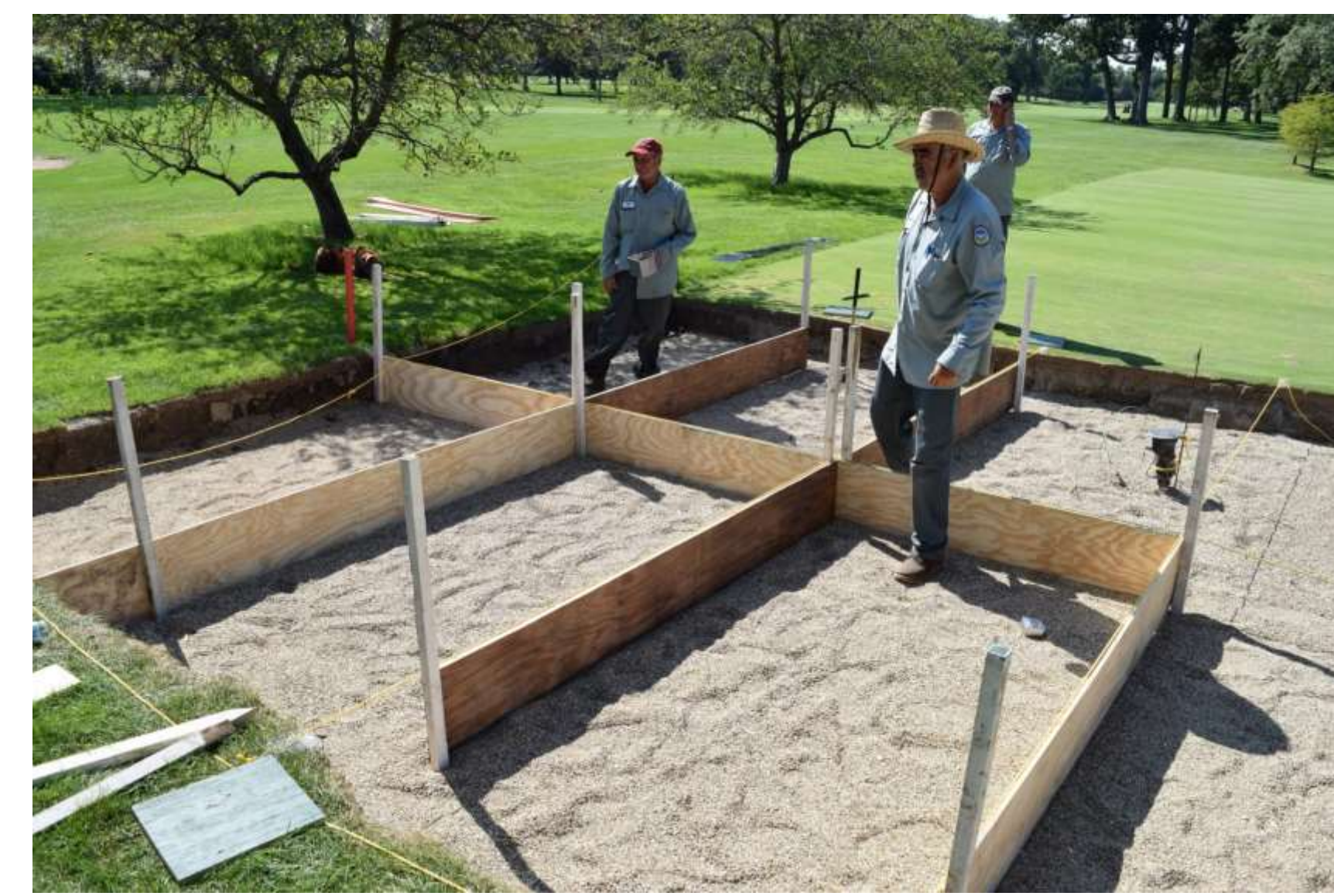
Fig. 1. North Shore CC staff building temporary plywood partitions.
